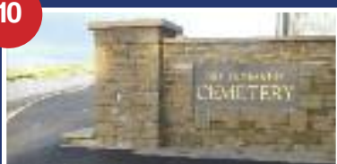
Building a new Dumbarton Cemetery in Garshake Road
