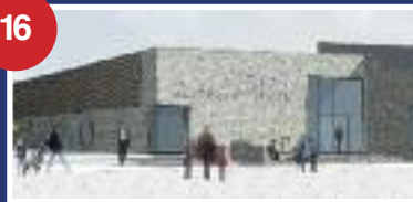
Building a new Kilpatrick Secondary School and centre
