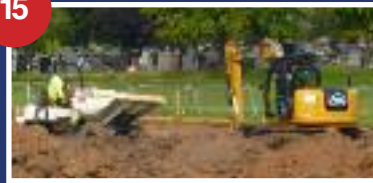
Upgrading Vale of Leven, Kilmarnock and North Dalnottar cemeteries
